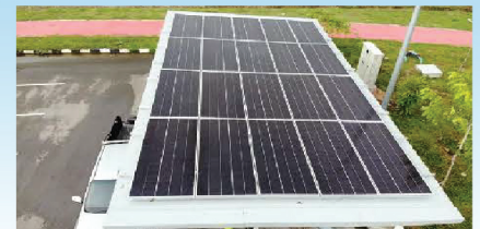
PV Solar Roof Top at Parking Lot for EV Shuttle Bus
