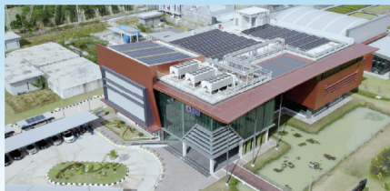
Microgrid at IOC Building (PV Solar Roof Top with Battery Storage)
